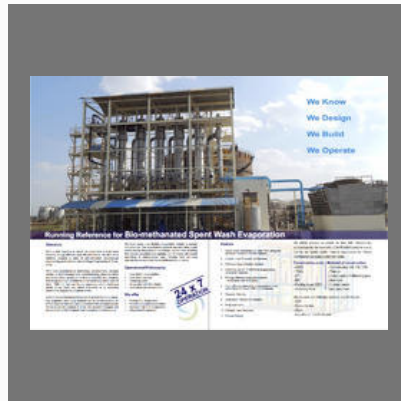
Spent Wash Evaporation
