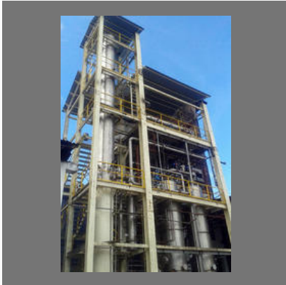
Fuel Ethanol Plant
